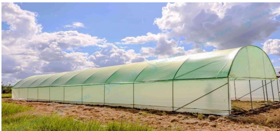
Figure28: Completed installed greenhouse
